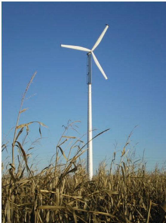
Entegrity Wind Systems 50kW turbine
