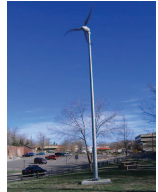
Skystream 1.8kW turbine
