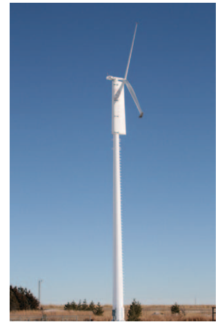
Entegrety Wind Systems 50kW turbine in Quinter, Kansas
