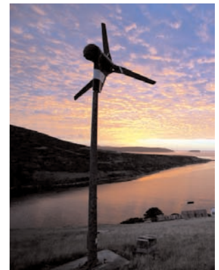
Proven Energy 2.5kW turbine
