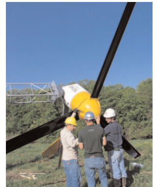
Bergey WindPower 10kW XLS turbine lowered for ground maintenance
