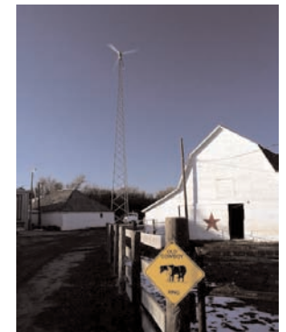
Bergey WindPower 10kW XLS turbine
