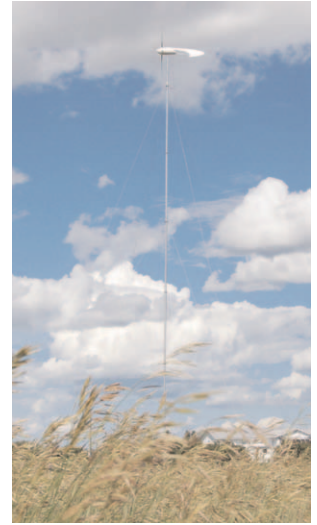
Windward Engineering 4.25kW turbine
