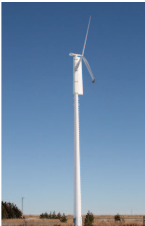
Entegrity Wind Systems 50kW turbine in Quinter, Kansas
